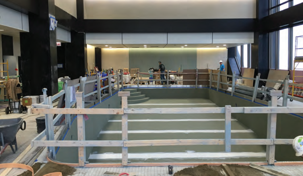
Pool and surrounding area under construction
