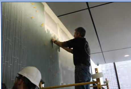
Wall tile installation
